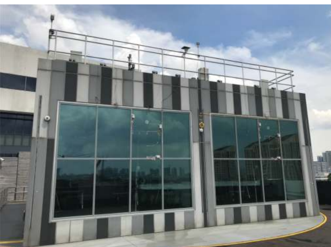
Conduct of experiment at BCA Skylab with thermally broken system on the left and non-thermally broken system on the right
