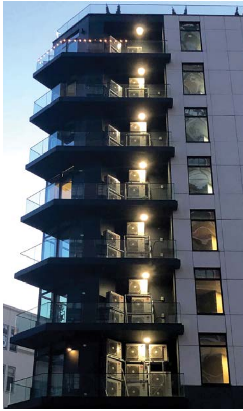
FIGURE 1: Challenges of heat pump deployment when heating loads are too high. PHOTO BY ENRICO BONILAURI, EMU PASSIVE
