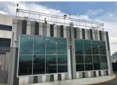
Conduct of experiment at BCA Skylab with thermally broken system on the left and non-thermally broken system on the right
